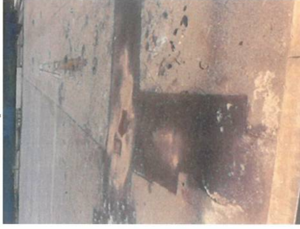
• Figure 2: Reinstatement asphalt
