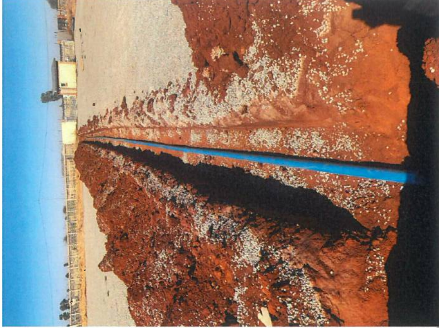
Figure 1: Fire reticulation being constructed
